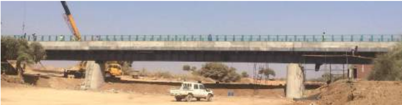
埃塞俄比亚DABOWEIN大桥 Ethiopia DABOWEIN Bridge 钢结吨位: 300余吨。 Steel structure tons: 300 tons 特点: H型钢梁简支梁三孔桥, 跨径为18.5+30.5+18.5米。 Features: H type steel beam bridge with 3 openings, span is 18.5m+30.5m+18.5m
