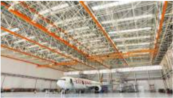
埃塞俄比亚机库 The Ethiopia Air Force Hangar 钢构吨位: 2939T Tonnage of steel structure: 2,939T
